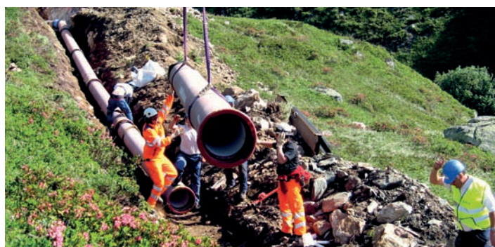
Laying in Alpine terrain
