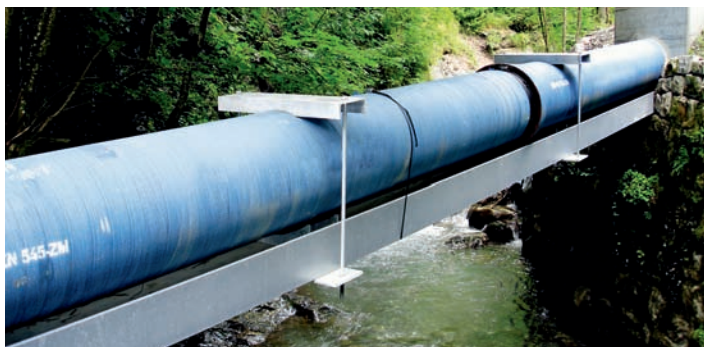
A pipe bridge
