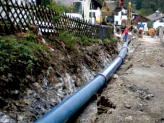
The run of pipeline just before the generator building
