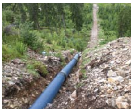
Laying work in rocky terrain
