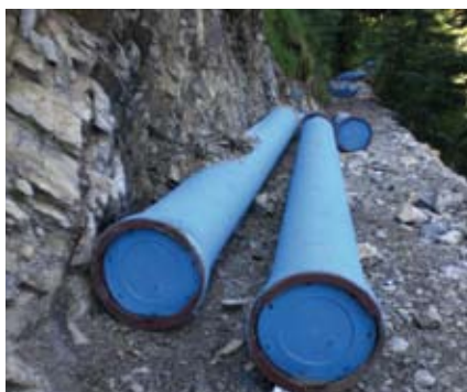
Laying work in rocky terrain
