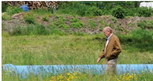
Wolfgang Rink, head of BGW's Applications Engineering Division, appraises the first section of the interim pipeline in the Hartenstein district.
