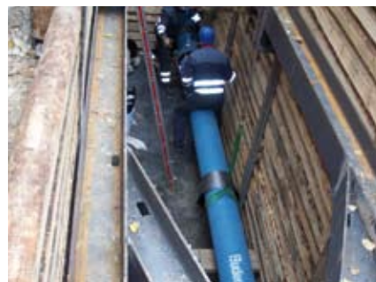
Installing the Buderus DN 300 ductile pipes
