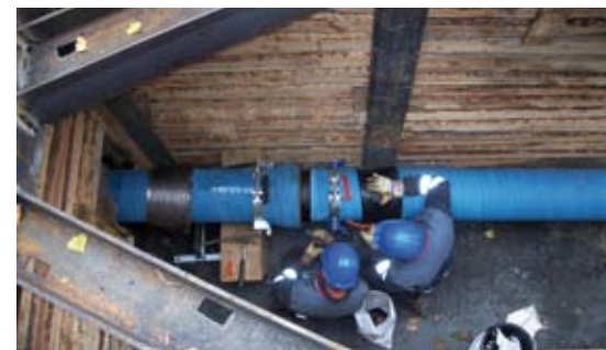
Making a BLS® restrained socket joint
