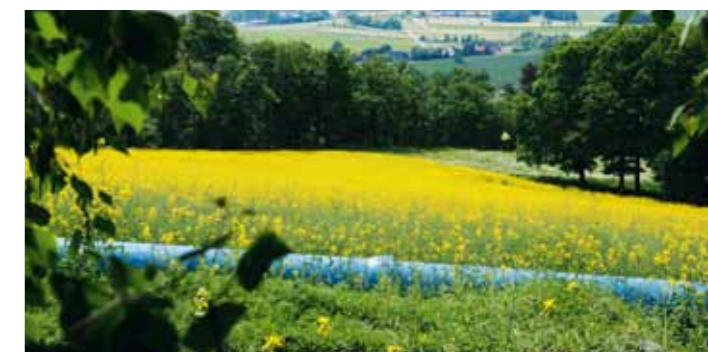
Temporary pipeline with BLS®-/VRS®-T joints
