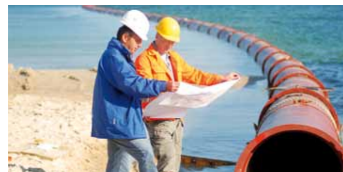
Floating in a ductile cast iron pipeline
